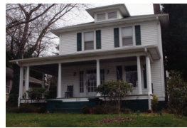
ROBERT J. MCCOLLUM HOUSE (1910) 220 Gloria Avenue HOME OF JEAN AND BEN JOHNSON
