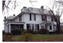
BURTON CRAIGE HOUSE (C. 1860/1928-29) 134 Cascade Avenue
